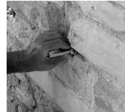
Figure 10: Tying with threaded bars
