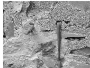
Figure 5: Leakage from a joint
