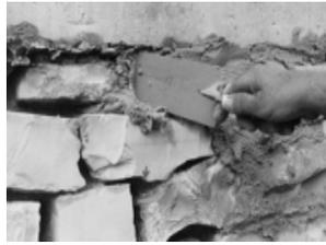
Figure 8: Filling of the joints with new mortar
