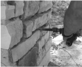
Figure 7: Mechanical excavation of the joints
