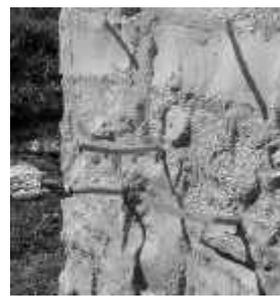
Figure 6: Leakage from an injection hose
