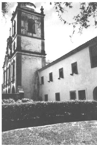
Figure 5: Impregnation of humidity on the external plasterwork.
