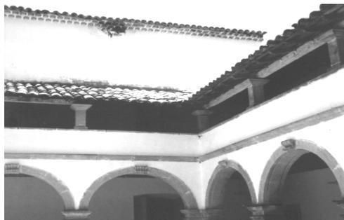
Figure 2 : Roof tiles cracks/ obstruction of drips causing infiltration.
