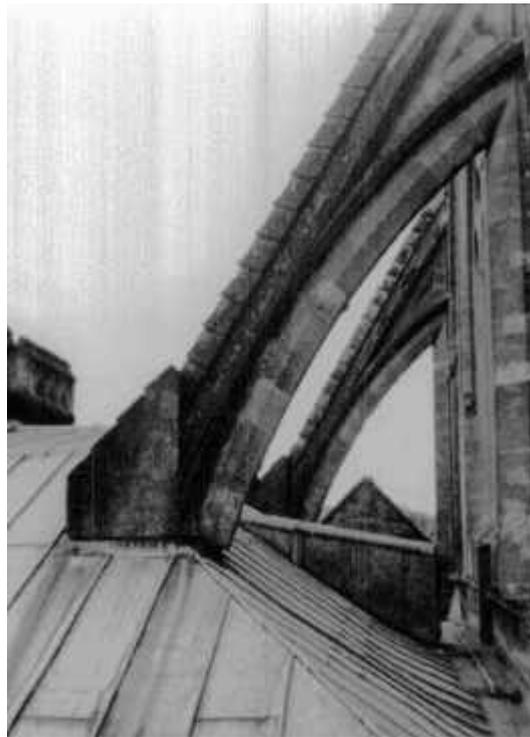
Figure 1 The Wells buttress above the roof
