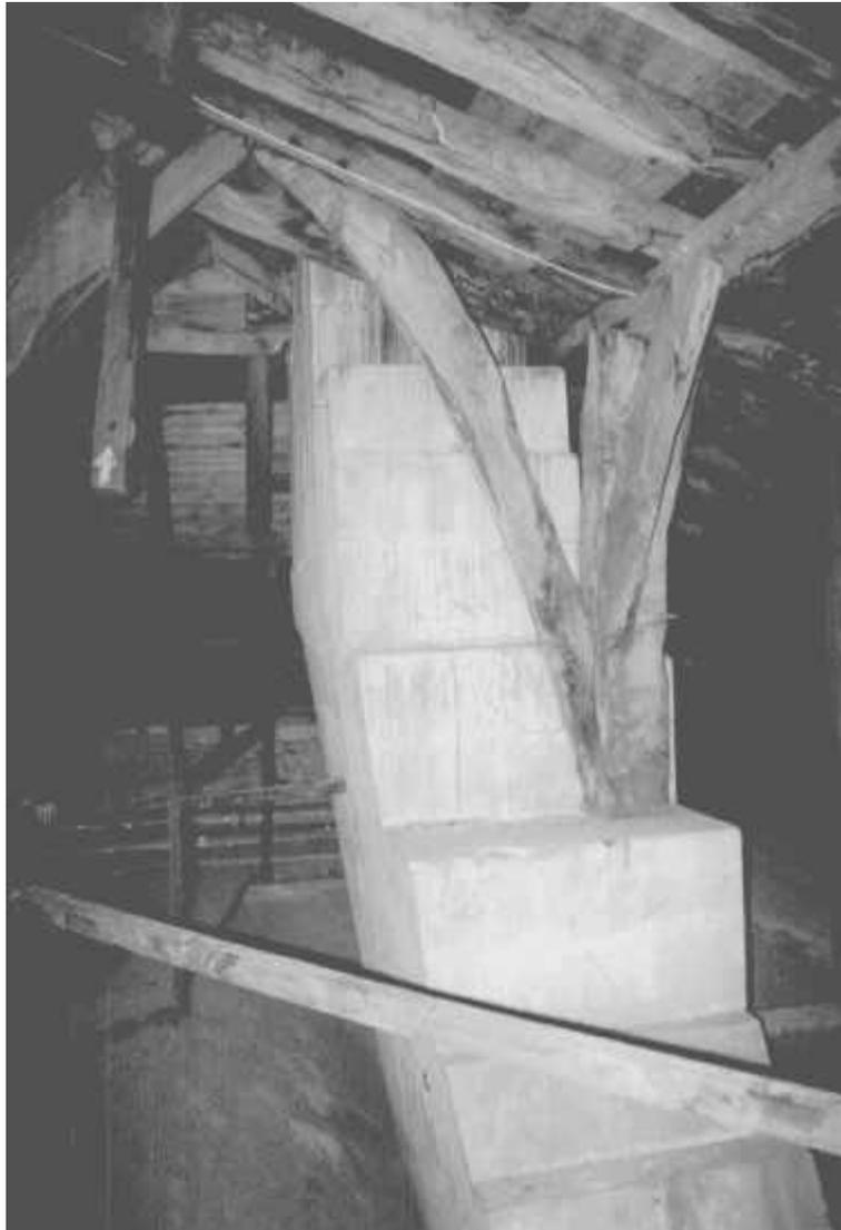
Figure 2 The buttress steps sideways in the roof space
