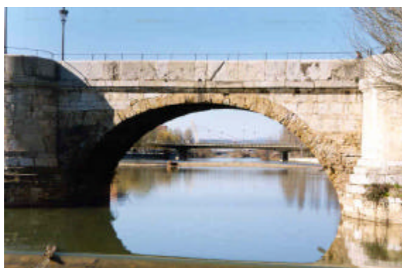
Figure 13: “San Marcos” bridge
