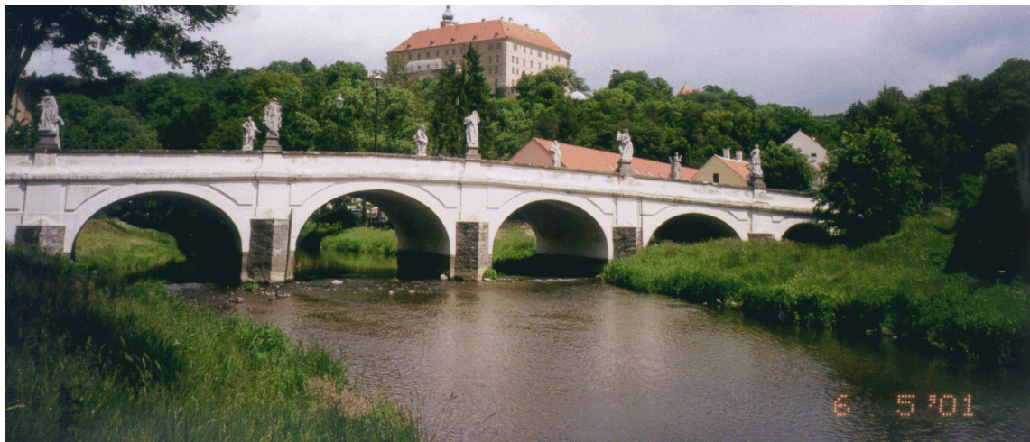
Figure 1 : The view of Náměšt nad Oslavou Bridge
