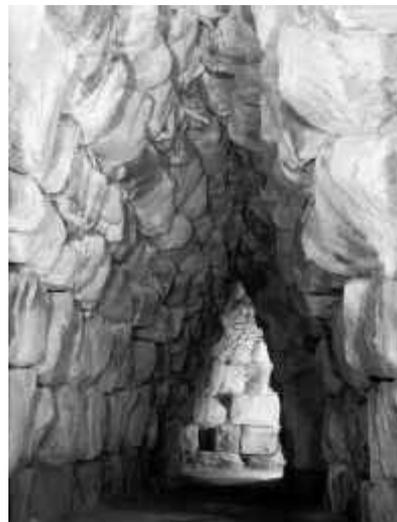
Figure 3: The stone vault of a corridor
