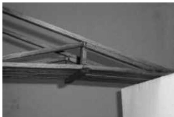
Figure 3 : View of a model of Palladio's Cismone bridge.
