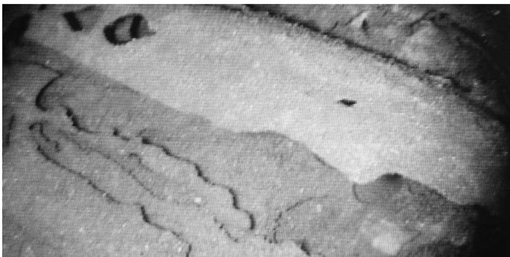
Figure 5 : Remaining parts of a collar beam inspected by videoscopy.
