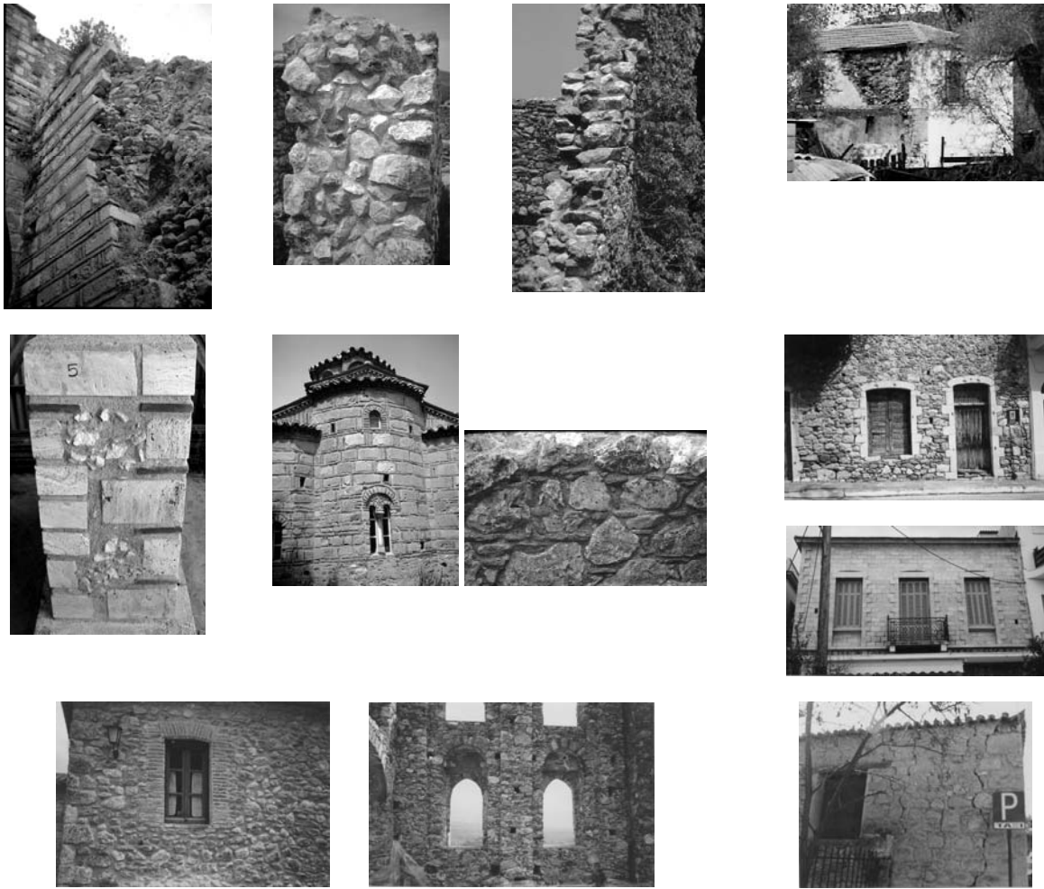
Figure 1 : Various types of masonry.
