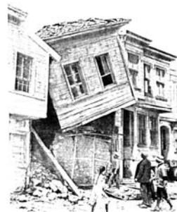
Figure 4: A damaged traditional timber frame house, in the Mürefte earthquake in 1912 (Cogito, 1999)
