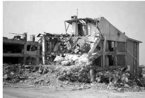
Figure 21 : A damaged reinforced concrete building after 1999 Düzce earthquake (Archives: Aşkun, İ. Y.)
