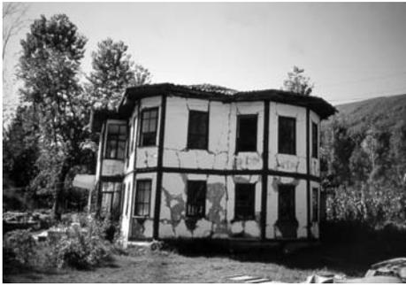
Figure 20 : An infilled timber framed house with a little damage after 1999 Düzce earthquake (Archives: Sezgin, H.)
