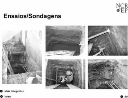
Figure 8 : In-situ probing of the foundations.
