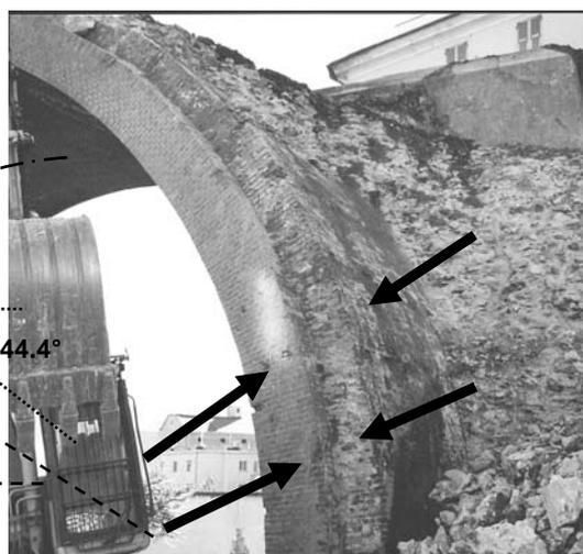
Figure 6 : *Cornigliano viaduct* (1932) during its demolition (June 2001): the barrel thickness is 65% higher than the external apparent value
