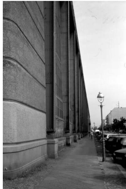
Figure 3 : AEG turbine fitting shop, longitudinal front with solid web stanchions
