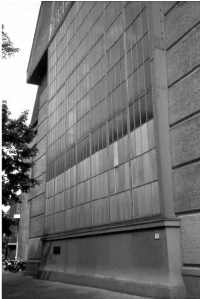
Figure 2 : AEG turbine fitting shop, footing with projecting base the nave front window
