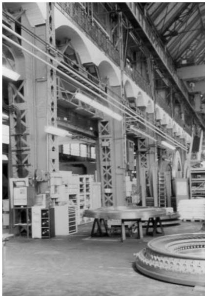
Figure 6 : AEG turbine fitting shop, view to the aisle gallery with reinforced concrete cellar vaulting and to the node of the roof truss tie rod
