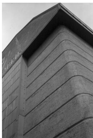
Figure 1 : AEG turbine fitting shop, nave end with front gable and window flanked by one of the battered reinforced concrete corners \*
