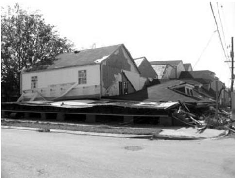
Figure 3a : This row of houses in New Orleans, were originally one story wood frame buildings. Termite damage caused one to buckle (left) at the lower level, causing all four to collapse in succession
