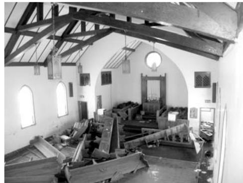
Figure 3b : In this historic church in New Orleans the water was 2 meters deep and was not drained away for a week. Three months after the storm, no clean-up had begun, leading to growth of mold and fungi.
