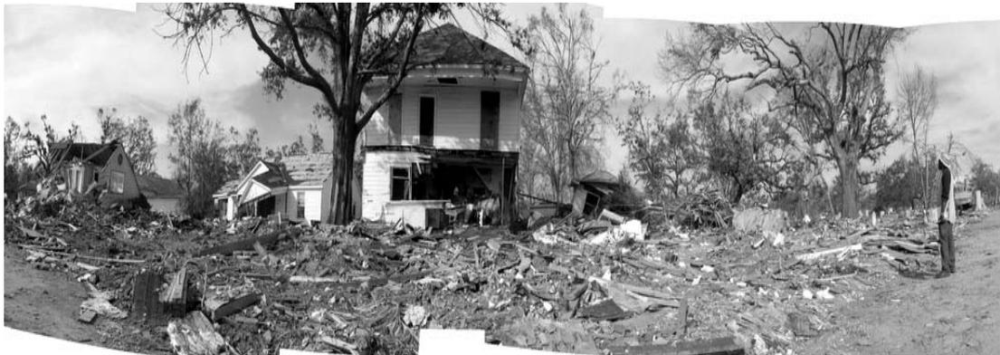
Figure 2 : A typical scene of destruction, west Gulfport, Mississippi, showing the debris field and first-floor damage to one of the few standing structures. A structural engineer (right) surveys the damage.
