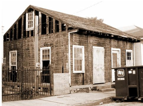
Figure 2 : Contemporary view of a *mardiers debout* framing technique on a building where clapboard siding is removed to reveal standing plank construction
