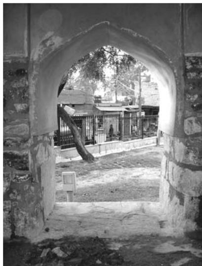
Figure 10 : Bara Khamba, Nizamuddin – Replastering of an arch has undermined its original proportions (Author, 2005)
