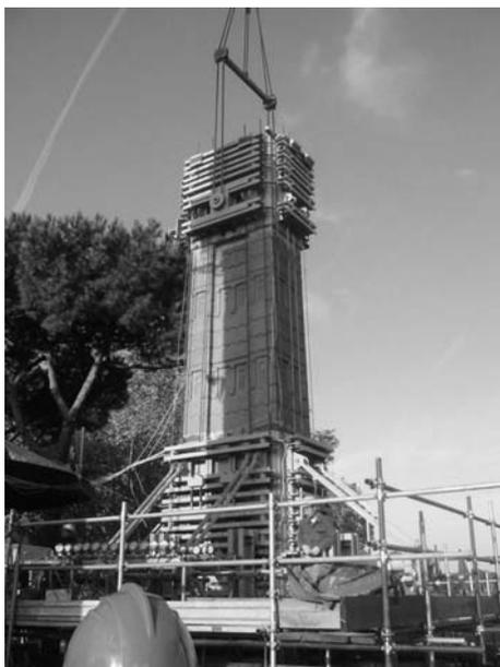
Figure 3 : Axum stelae in Rome, disjointing operation
