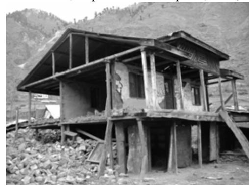
A timber house with Dhajji Dewari in Azad Jammu and Kashmir that survived the 8th Oct 2005 South Asian Earthquake (note: external stone walls collapsed).
