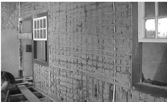
Figure 1 : Lath-and-plaster wall, Casa da Baronesa, Ouro Preto - State of Minas Gerais (Source: IPHAN’s collection).
