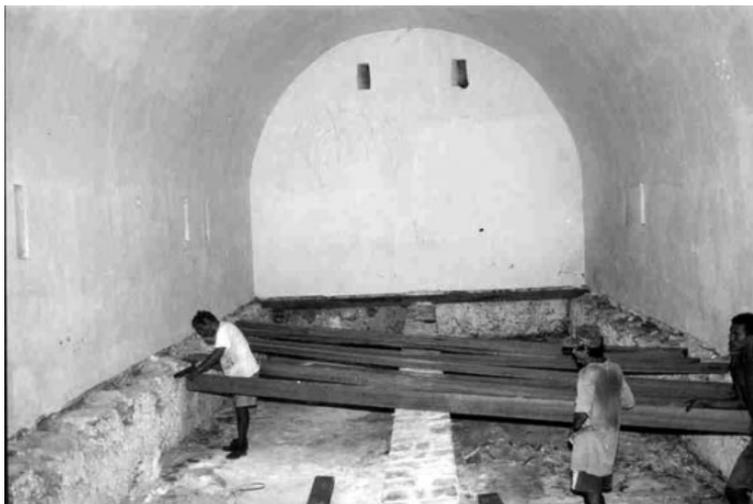
Figure 4 : Air chamber under the floor, Magazine, Fort São José de Macapá - State of Amapá (Source: IPHAN's collection).
