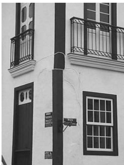
Figure 8 : Reintegration of coating cavities, Centro Cultural da FIEMG, Ouro Preto - state of Minas Gerais (Source: IPHAN's collection).
