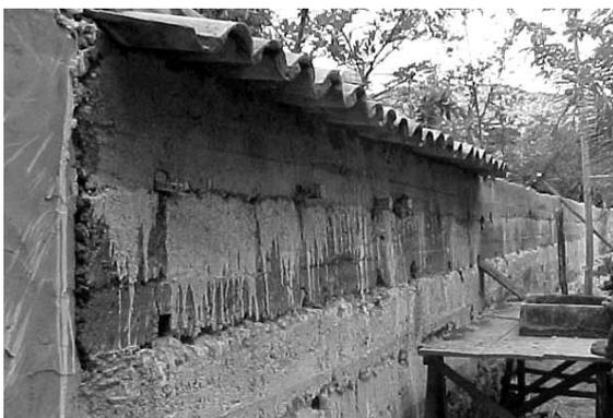
Figure 3 : Rammed earth wall under rebuilt, Casa Cora Coralina, city of Goiás - State of Goiás.
