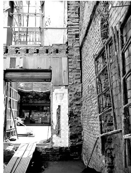
Figure 3 : Dividing fence fastened to façade in Menéndez Pelayo Avenue 23
