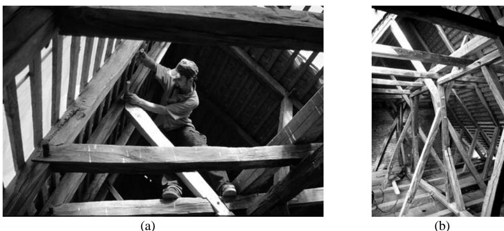
Figure 8 : The restoration of the roof structure of the Unitarian church in Maiad – Mures: (a) completion of missing element (b) overall view of the restored roof
