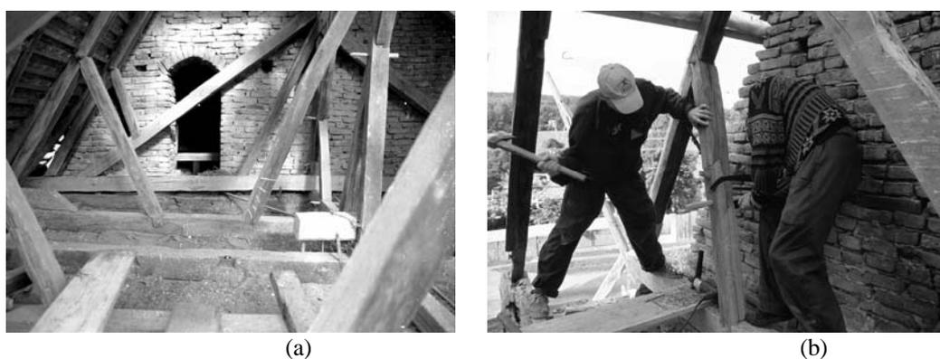
Figure 7 : The restoration of the roof structure of the Unitarian church in Maiad – Mures: (a) element partially eliminated during previous consolidation works and (b) completed element
