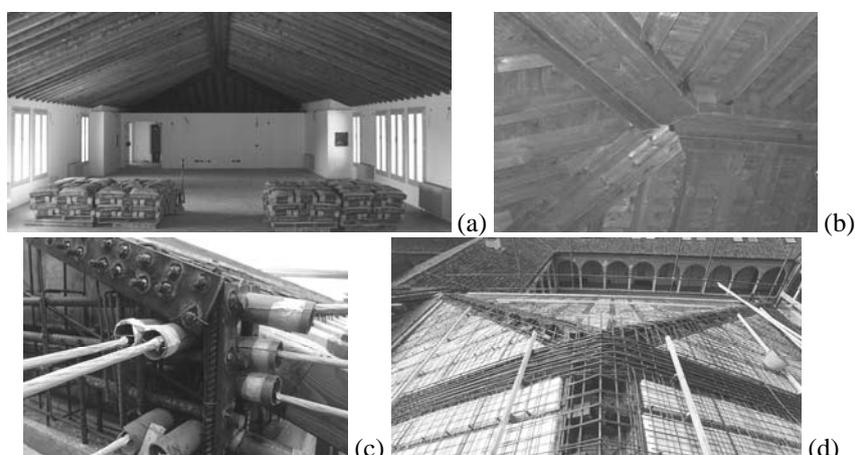
Figure 9 : Santa Chiara Building: (a,b) internal views of the roof structure; (c) detail of the ordinary rebar of the eaves chords and head of the prestressed rebar; (d) detail of the hipped end.
