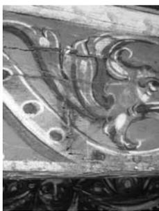
Figure 6 : Deflection breakage
