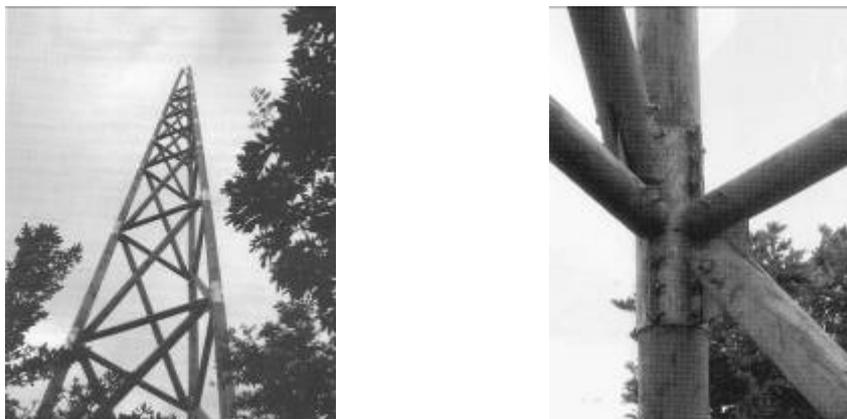
Figure 7 : Uniform round timber communications tower and joint detail
