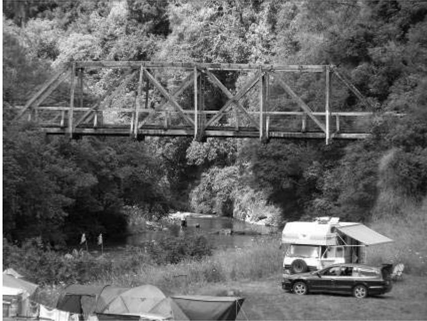
Figure 4 : Manganuku Stream Bridge, Howe truss structure
