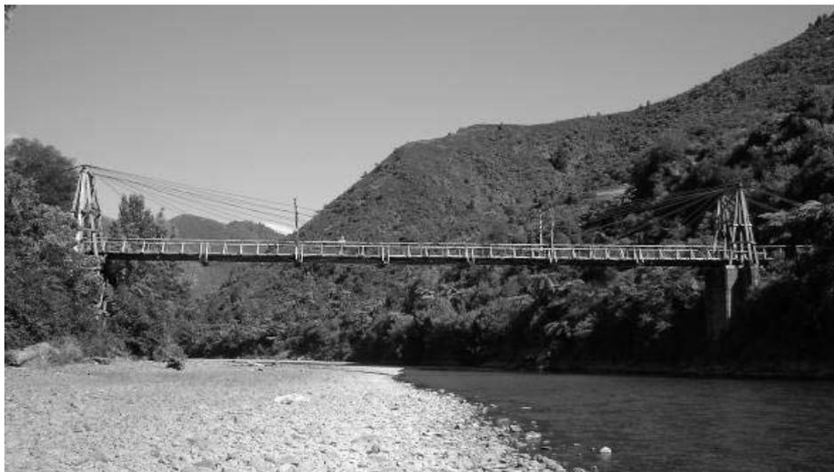
Figure 1 : Tauranga Track Bridge, harp suspension structure.
