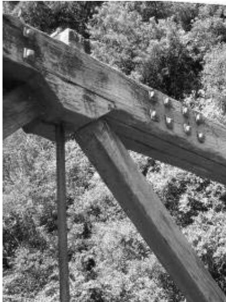
Figure 5 : M.S.B., top chord joint
