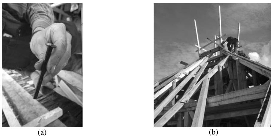
Figure 7 : (a) The shingles were attached with flat forged nails. Driven in crosswise, they break the grain of the wood nut do not split the shingle; (b) The roof structures were assembled partly with rowan wood pegs and partly using hand forged iron tie rods and bolts.
