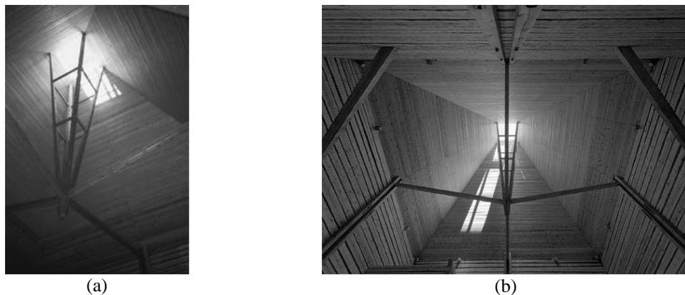
Figure 9 : (a) The only window in the church is the lantern skylight in the roof. The visible structure of the upper part of the church consists of eight long beams; (b) The horizontal beams bear the outer walls and the vertical beams of the roof. The joint is made of wedges so that it is flexible.
