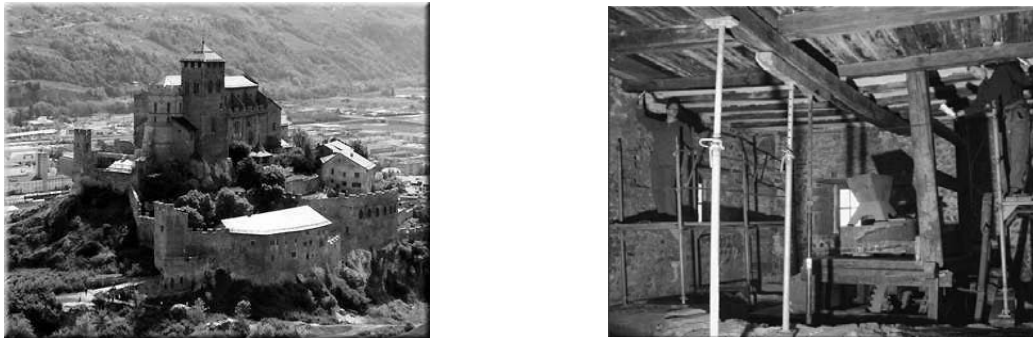
Figure 9 : Valere's Castle, Sion, Switzerland, built during the XIIIth century. Non-destructive evaluation of the wood residual strength by using Sylvatest-Duo.
