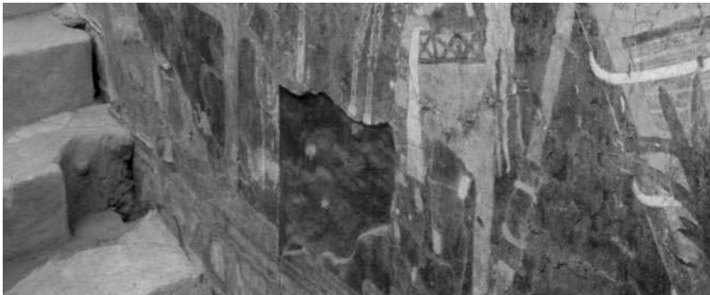
Figure 2 : Typical detachment of a segment.
