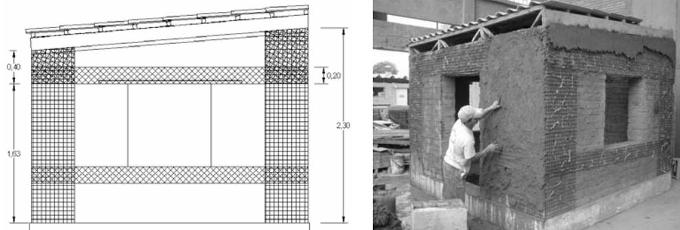
Figure 9 : Reinforcement arrangement and construction of model M050-T11.
