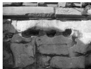
Figure 17 : Broken sandstone at the outer enclosure.
