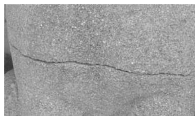
Figure 7 : Cracks at the base of the column.
