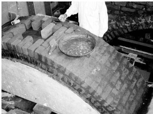
Figure 3 : Construction of arch barrel in progress.
