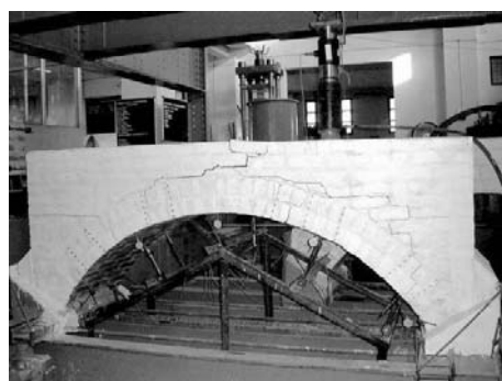
Figure 8 : Cracks in the arch barrel and the spandrel wall in AF2 arch.
