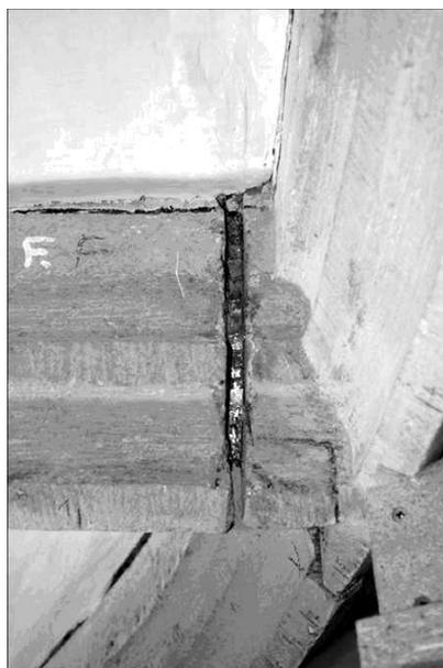
Figure 4 : repaired historic lead joint in a reticulated vault. Here, the lead stops before the lower fillet to prevent excessive edge pressure.
