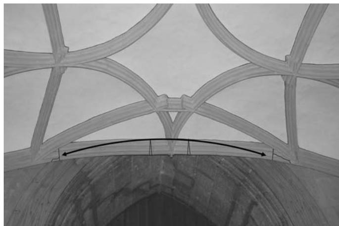
Figure 2 : Deformed arch of the gallery vault with the resulting thrust line. Seen from below, looking West
