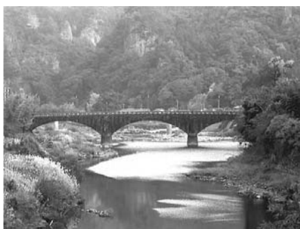
Figure 1 : Rakanji stone arch bridge
