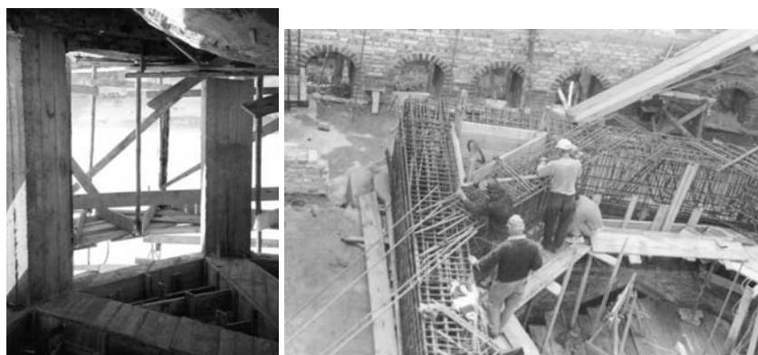
Figure 12 : Central tower construction and reinforcement of the tower base-raft structure.
