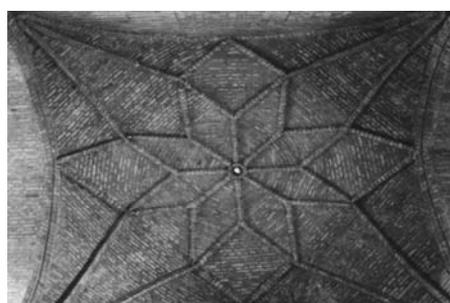
Figure 13 : Details of stellar gothic vault after reconstruction.
