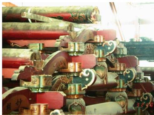
Figure 2 : Small structural components forming the upper part of Dieh-Dou structure by stacking and mortise tenon connections. (photo taken by Chow).
