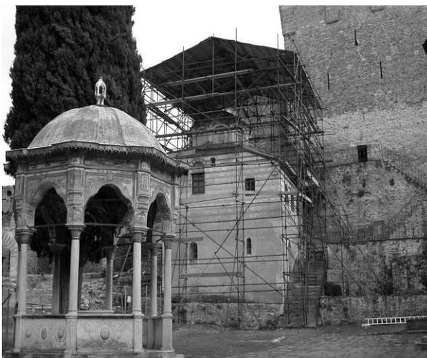
Figure 7 : Protective construction over Paraclis of Holy Archangels,
