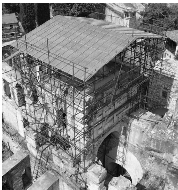
Figure 8 : Protective construction over Paraclis of St. Nicolas Church,
