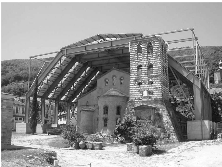
Figure 10 : Protective construction in The Protat Church, Carea
