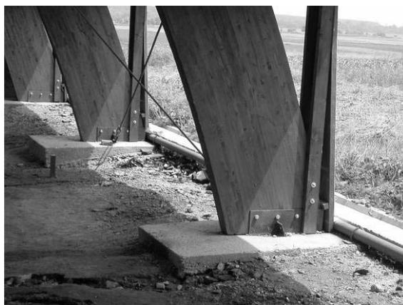
Figure 2 : Connection of the bearer with the footing, protective construction over Roman bath, Viminacium
