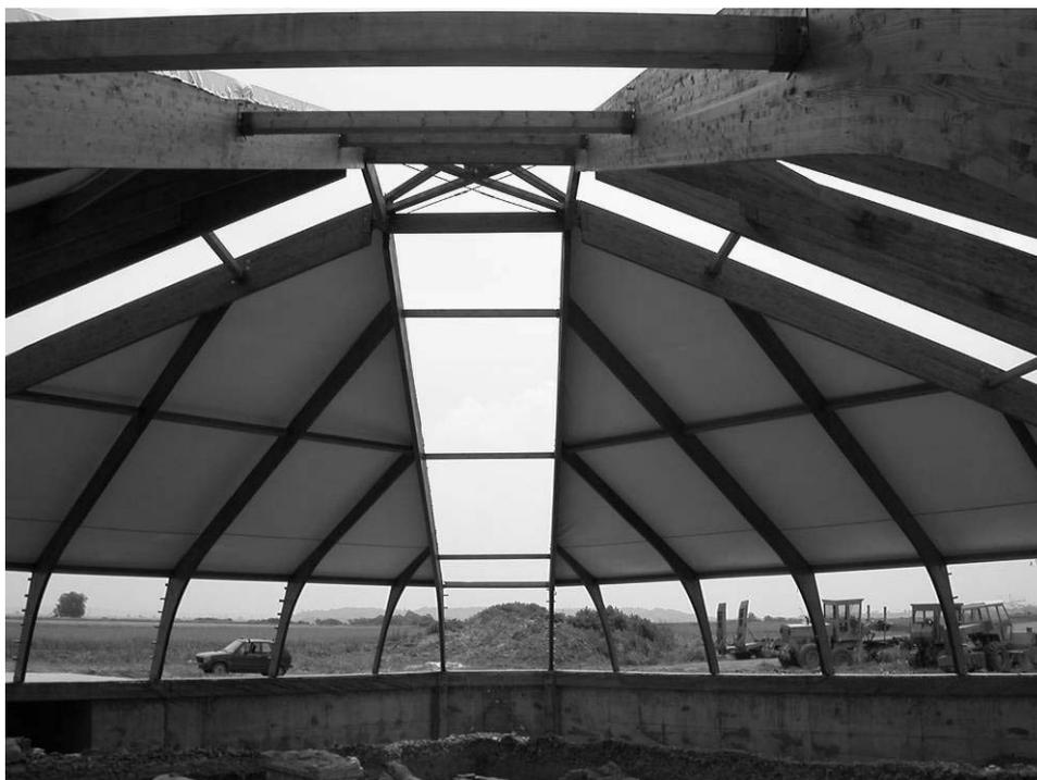
Figure 3 : Pyramidal protective construction over the graves, Viminacium
