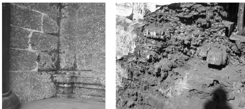
(a) Efflorescence due to deposition of salts on surface      (b) Progressive damage due to deposition of salts internally
