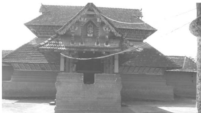
Figure.3 : Typical traditional temple in Kerala built using exposed laterite masonry.
