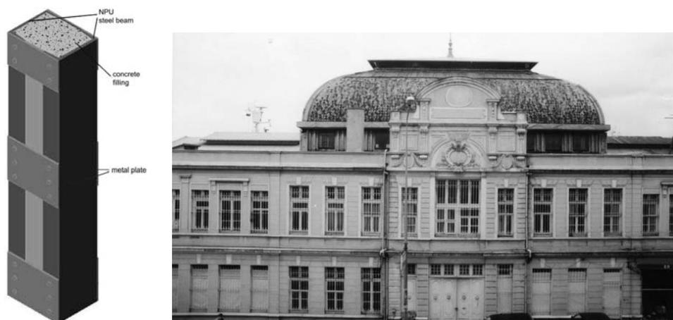
Figure 9-10 : Iron-concrete construction technology. Galata Customs Building (1907), one of the first buildings constructed with iron-concrete construction technology (U.Yergün).
