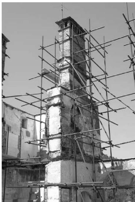
Figure 6 : Protection of walls with a tube-shaped scaffolding
