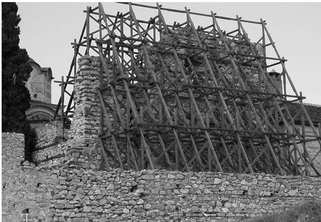
Figure 1: Protection of wall of stone with a wood truss, St. Vasilije
