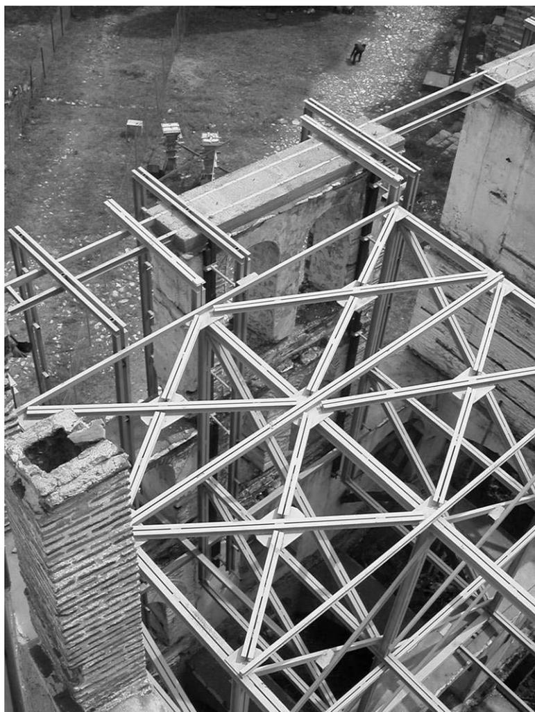
Figure 4 : Spatial construction for protection of walls
