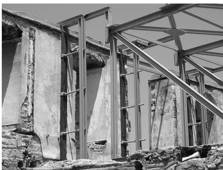
Figure 5 : Way of supporting the walls
