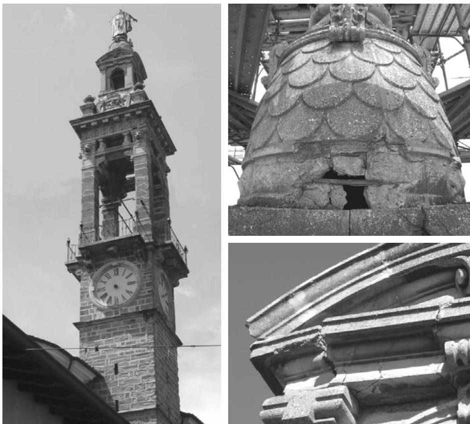
Figure 1 : View of the St. Sisto's bell-tower and particular of the damages induced by the impact of lightnings against the walls.
