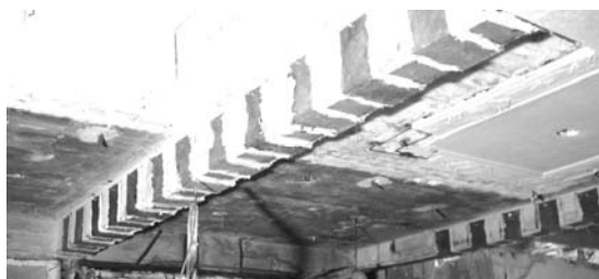
Figure 11 : Strengthened beams in Bank of China
