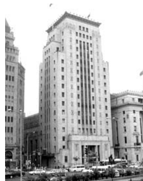
Figure 2 : Bank of China
