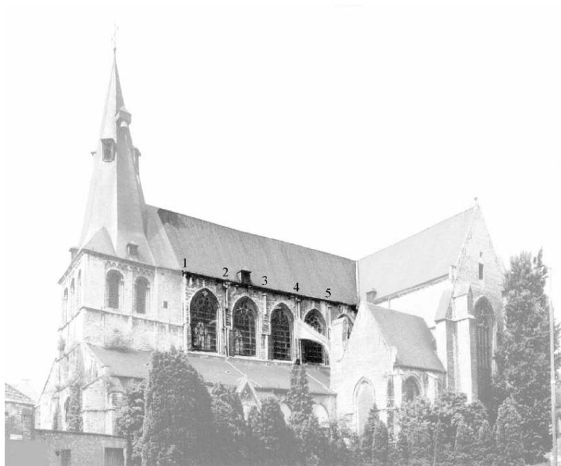
Figure 1 : South Facade, with the 15<sup>th</sup>-16<sup>th</sup> century alteration emphasised
