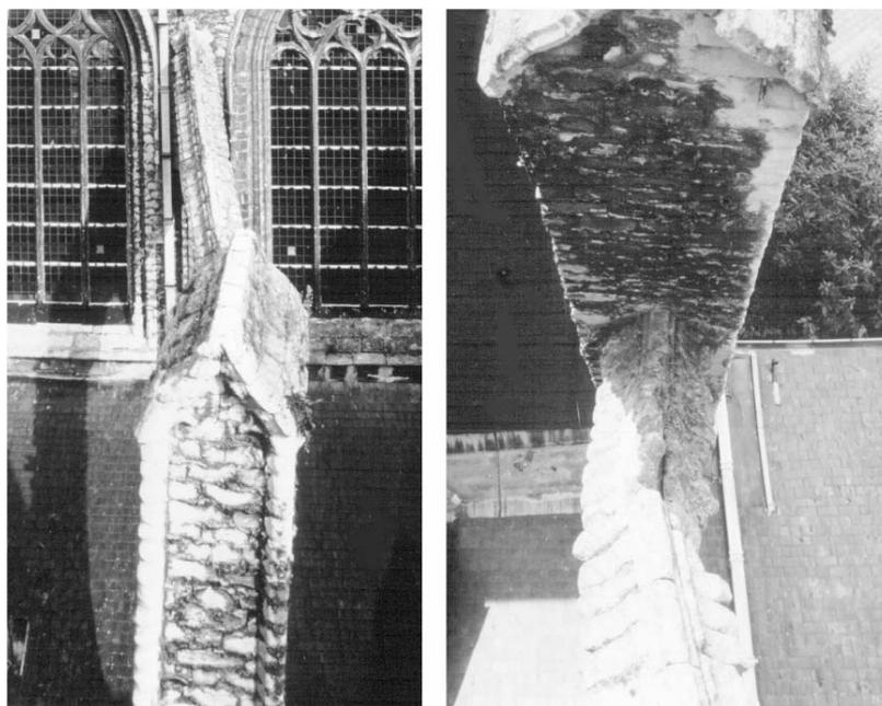
Figure 2 : South-Western flying buttress (FB-4S). Left: misalignment of the structural elements. Right: view from the top of the angled bend in the arch, near the buttress
