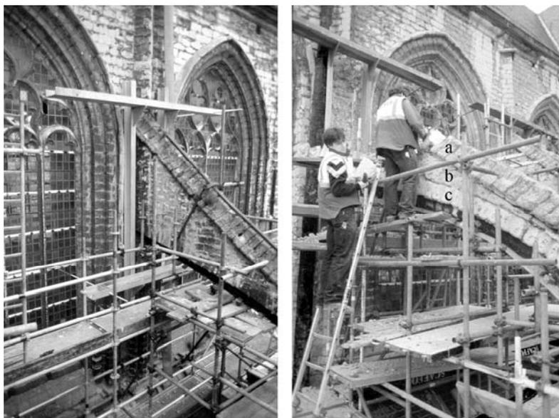
Figure 3 : South facade, dismantlement of the South-Western flying buttress (FB-4S).
