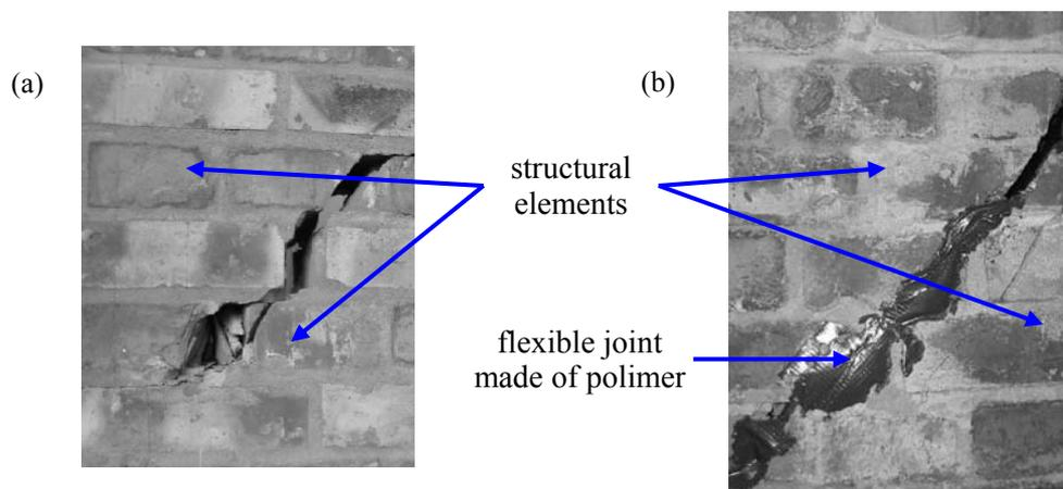
Figure 1 : Application of the Flexible Joint Method: (a) cracked masonry wall, (b) flexible joint made of polymer, filling in crack and joining disrupted structural elements.
