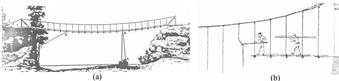
Figure 1 : (a) Experimental bridge designed by Seguin; (b) Constructive process of a wire bridge (Wagner 1993) as related by (Dufour 1824).
