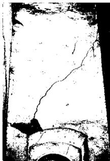
Figure 5 : Crack on the wall of the mezzanine floor.
