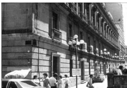
Figure 1 : Great distortion of the old School of Mines without visible cracking in stone masonry
