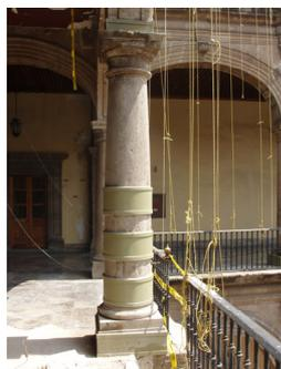
Figure 8 : Confinement with steel plates of a damaged arcade column
