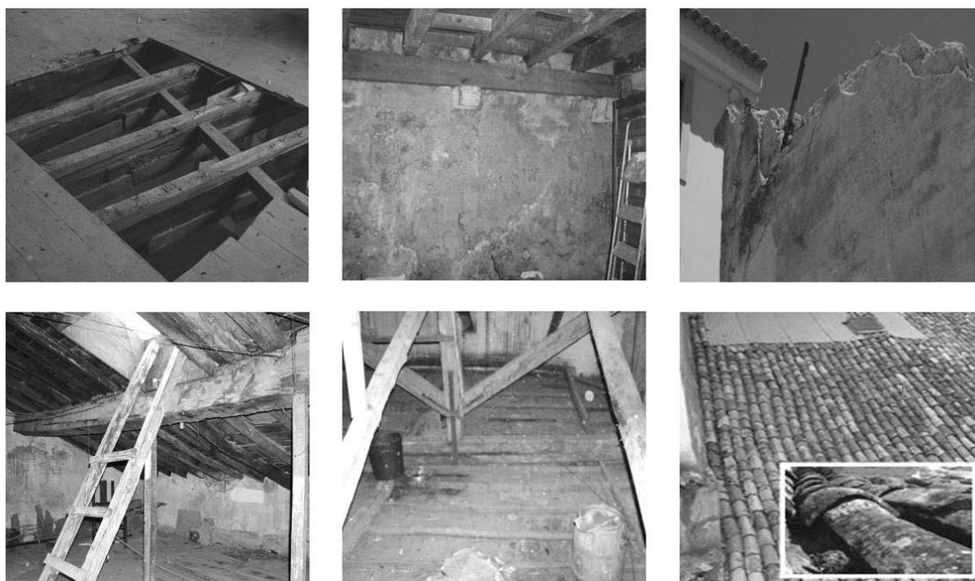
Figure 4 : Timber floor and roof structures
