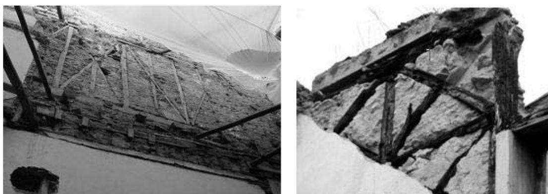
Figure 3 : Timber triangulated structure
