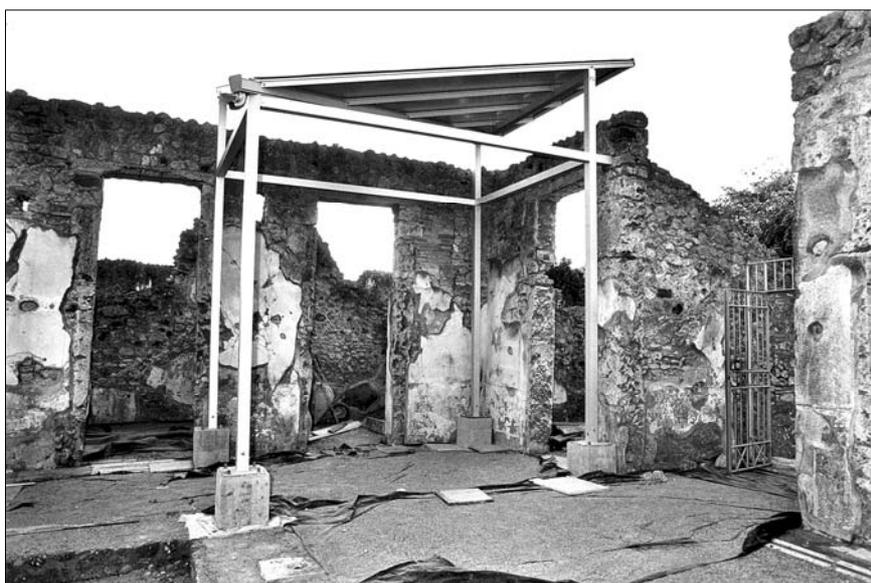
Figure 4 : Prototypal cover of a portion of the main atrium.
