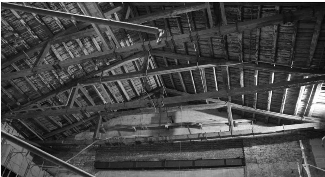
Figure 3 : The queen-post timber truss.
