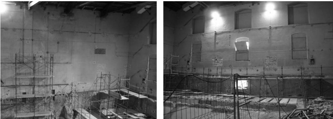
Figure 2 : The southern wall of the fly tower (note in the lower part free of plasterwork the discontinuity between the 18<sup>th</sup> century and 17<sup>th</sup> century walls); the western wall of the fly tower (note the openings in the wall, besides the three big arches not in view, in the lower part under the stage).
