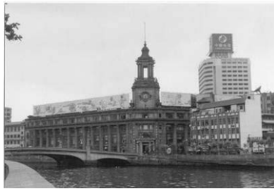
(a) South elevation view before strengthening
