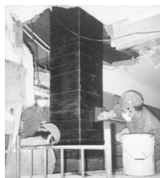
(b) Column strengthening construction
