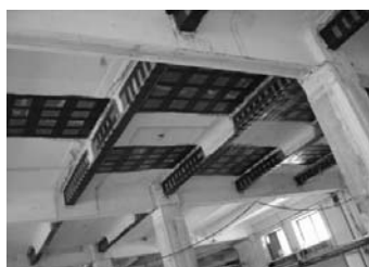
(a) Beam & slab strengthening construction
