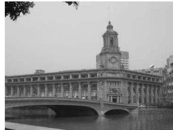
(b) South elevation view after strengthening
