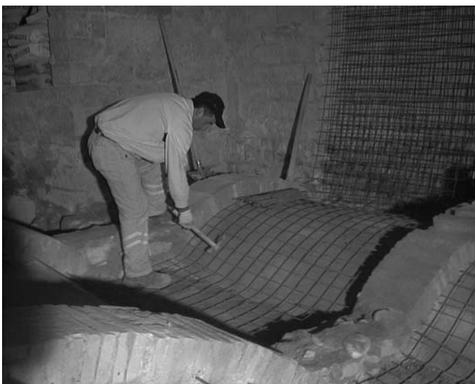
Figure 6 : Ground floor: reinforcing works
