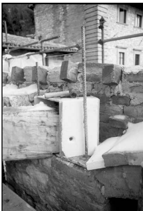
Figure 11 : Connection between roof beams and façade
