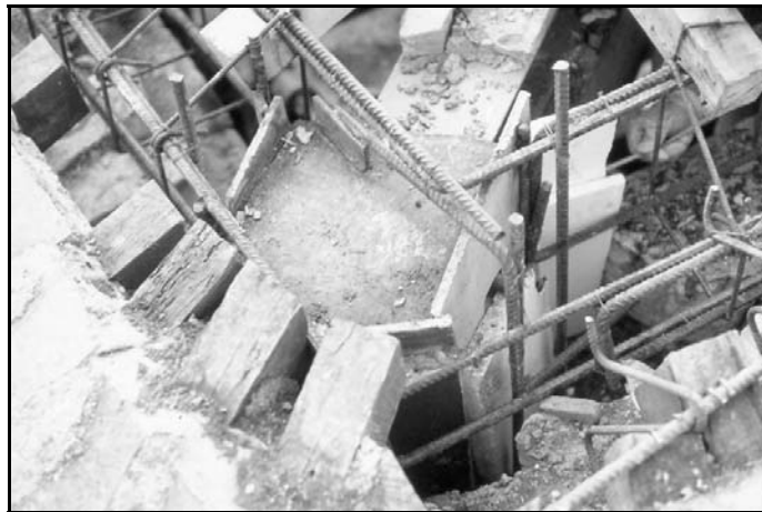
Figure 10 : The roof level
