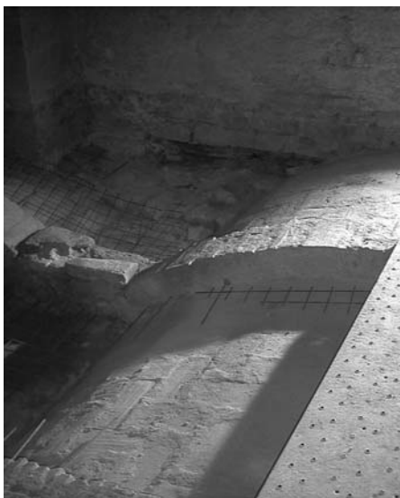
Figure 5 : Brikvaults reinforcing works
