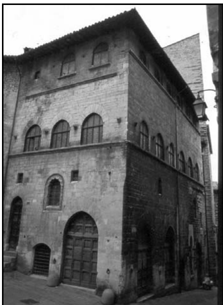
Figure 13 : Bargello Palace before the restoration
