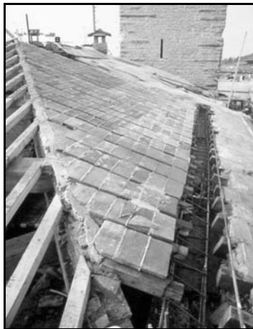
Figure 9 : Anti-seismic adjustment works
