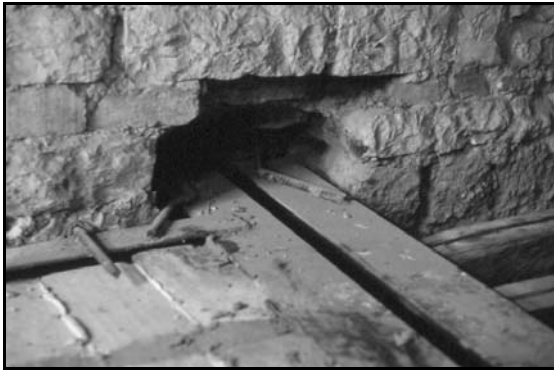
Figure 7 : Steel pins of the beams in the wall
