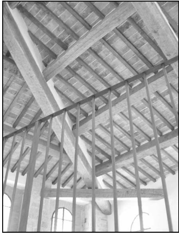
Figure 16 : the restored wooden covering structure
