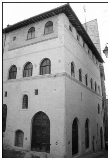
Figure 14 : Bargello Palace after the restoration
