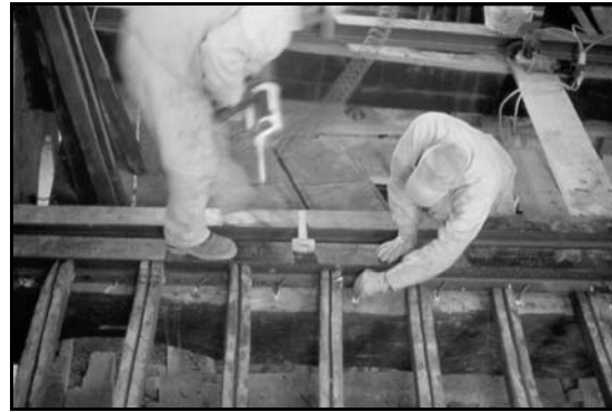
Figure 8 : Wooden floors' structure restoration
