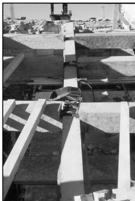
Figure 12 : Reinforcing on the extrados surface
