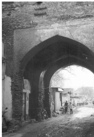
Figure 3 : Raj pura Gate Flooded almost every year. Dilapidated lower portions are visible.
